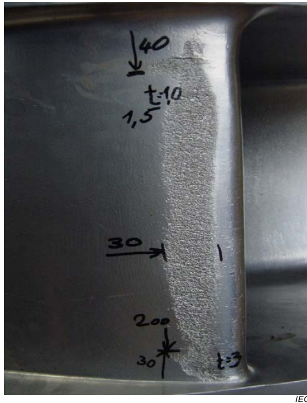
Figure 15 – Leading edge cavitation erosion on a Francis pump-turbine caused by extended periods of operation at very low loads
